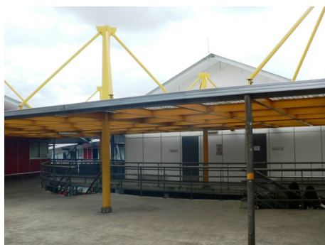
Replacement of fibreglass roofing
